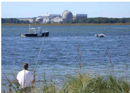
Seabrook Station Nuclear Power Plant in Seabrook, New Hampshire.
