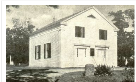
"Old Indian Meeting House," built in 1684 in Mashpee, is the oldest surviving Native American church building in the United States
