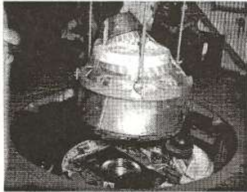
Figure 9. Installation of the MIDAS 6 Series III Infrared Sensor Payload atop the Agena B at PALC 1-2, November 1962 (note the spin table interface).
