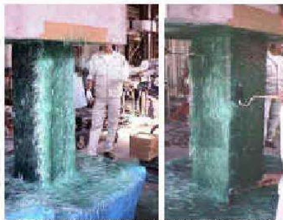
Photo 1. Construction site of sprayed-up FRP
